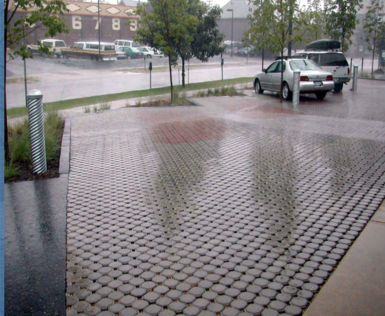
Permeable pavers allow water to infiltrate.
