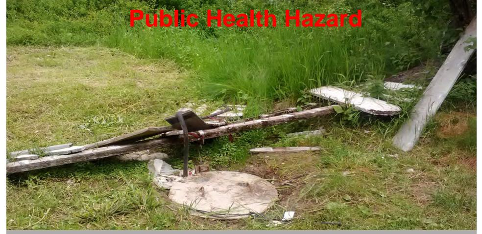
The drainfield is saturated and cannot accept wastewater. A hose & pump are being used to <u>discharge untreated wastewater from the septic tank directly into the</u> <u>wetland/creek.</u> This is a Violation of IDAPA 58.01.03. **System has Failed. Repair Permit Required.**  **CLOSE TO HOME**
